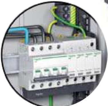
Surge arrester iPRD 4P + iC60N 4P
